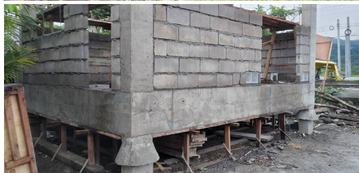
Phases of construction of the rice storage. Top photo: The structure made use of wooden scaffolds to construct the columns and elevated concrete slab. Bottom photo: The structure also used concrete hollow blocks for its walls and rat guards have been integrated in the reinforced concrete columns. Photo from RWAN.
