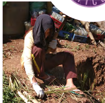
A community member planting vetiver along the eroded part of the road.
