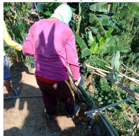
A community member compacting the soil on the first tier of the embankment.
