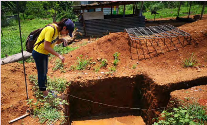
YP intern Anna Rienton checks the depth of a footing during a construction monitoring visit in MASAGANA community.
