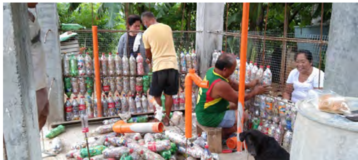
Community members of Masagana work together to build the wall of their multi-purpose community facility which is made of ecobricks.
