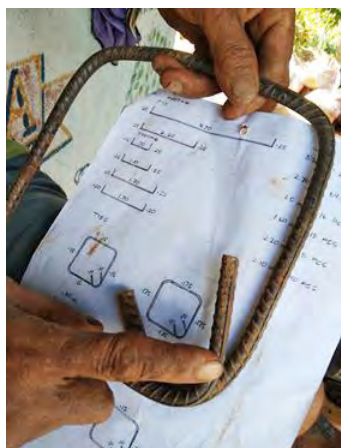
A worker asks about the ties to be used for the column of the multipurpose community facility (MCF).
