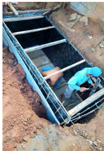
The workers secure the formworks for the cistern prior to concrete pouring. (Photo credit: Masagana)
