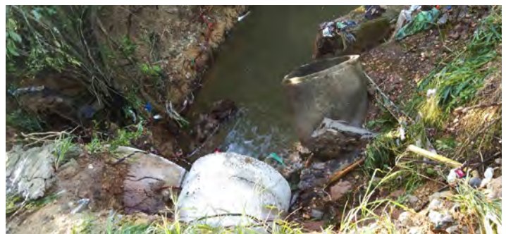
The concrete pipes along with some of the soil were moved by the flow of water. (Photo credit: Masagana)
