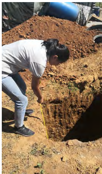
Dessica Salvador measures the depth of a footing excavation during a site visit in Masagana just before the enhanced community quarantine.
