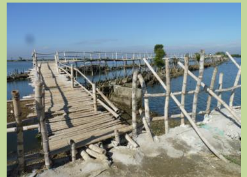
Left: SAMASAISIP community members, mostly fisher folks, drive bamboo poles into the fishpond; Right: Bamboo poles form a ramp to reach the elevated walkway.
