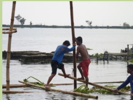
Left: SAMASAISIP community members, mostly fisher folks, drive bamboo poles into the fishpond; Right: Bamboo poles form a ramp to reach the elevated walkway.
