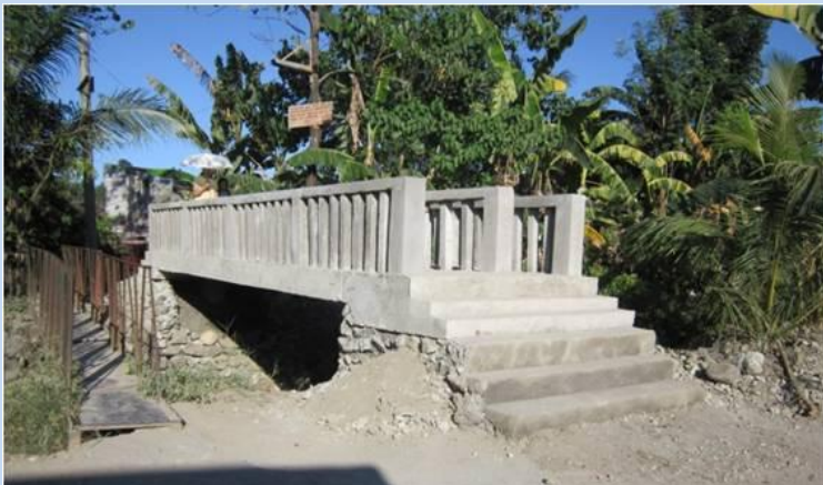
Top: Steel reinforcements for the concrete bridge to ensure earthquake-resilience. Bottom: The completed pedestrian bridge that connects Phase 1A and Phase 1B of Suburban; at left of the concrete bridge is the existing metal bridge that residents have been using to cross the area.
