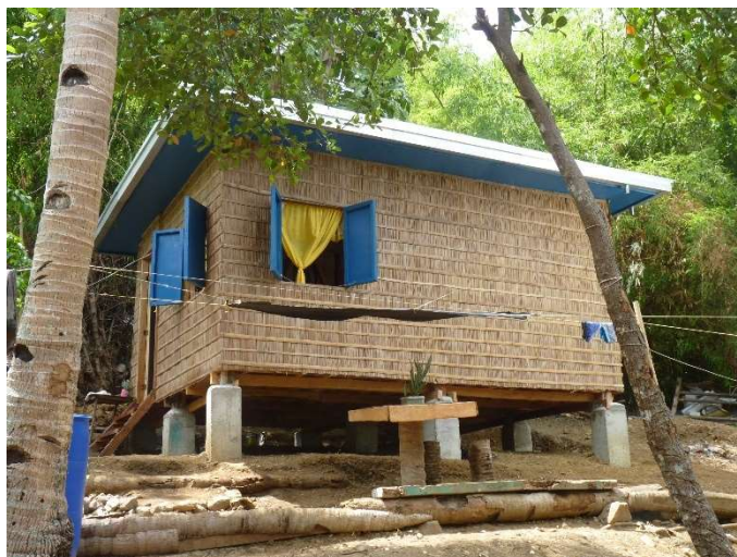
Typical design of transitional shelter in Punta Buri, with raised flooring and concrete pedestal
