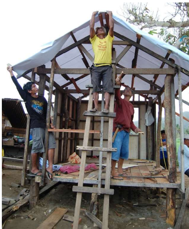
Local carpenters from Mapanas build a transitional shelter using the emergency shelter kit
